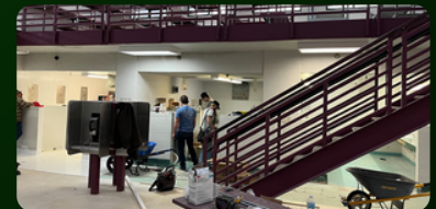
Housing Unit Repairs
