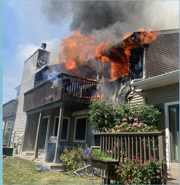
18 different area fire agencies responded to the 2022 fire pictured above.
