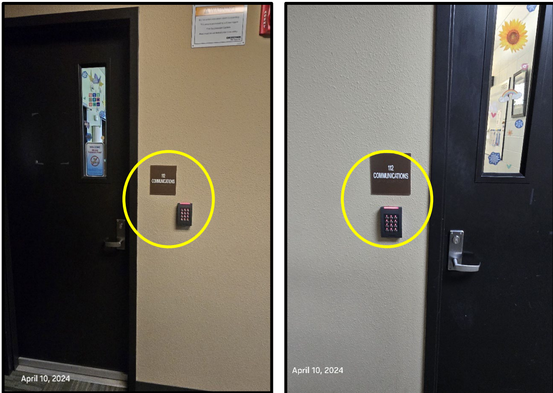
Figure 12: Door Entrance Points Leading into the ECC
