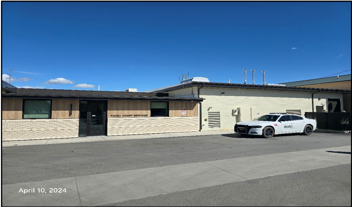
Figure 27: Exterior View of Back-Up Facility (Front)
