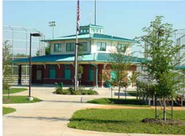
Central concession/pressbox and restroom building
