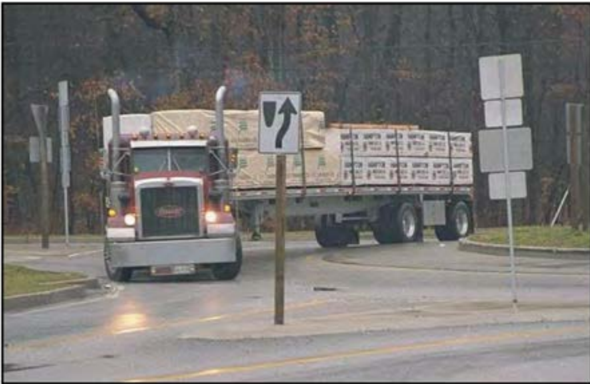
LARGE TRUCK OVERTOPPING THE TRUCK APRON
