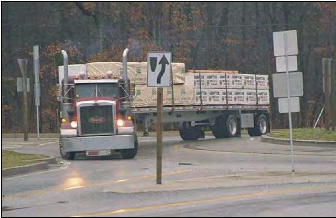
LARGE TRUCK OVERTOPPING THE TRUCK APRON
