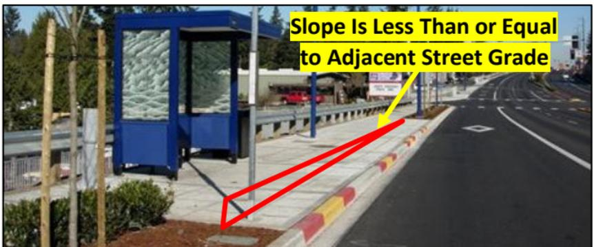
Figure 86: Slope of Boarding and Alighting—Parallel to Street
