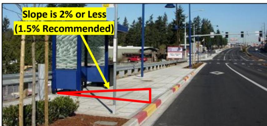
*Figure 87: Slope of Boarding and Alighting Areas—Perpendicular to Street*
