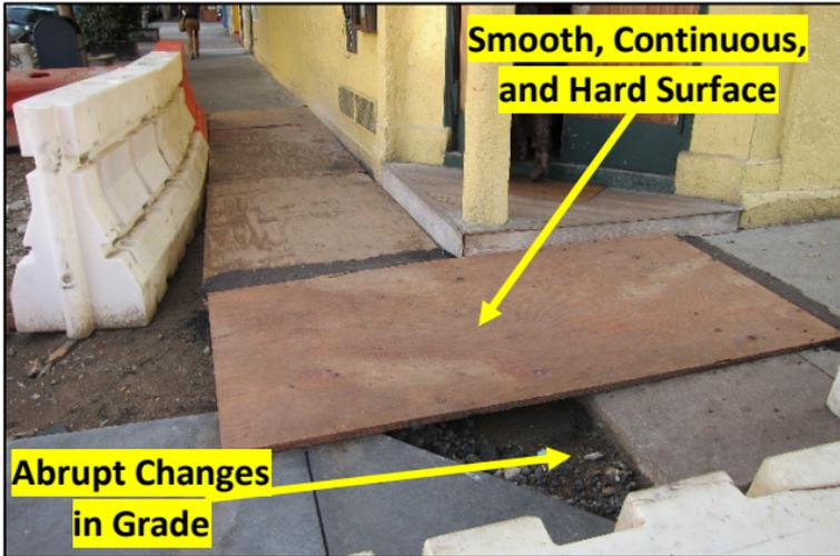
Figure 29: APAR with Abrupt Grade Changes and Treatment
