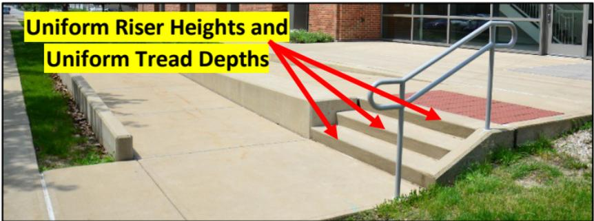
Figure 109: Uniform Riser Height and Tread Depth
