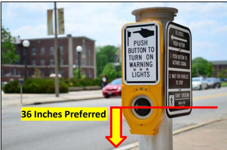
Figure 80: Pedestrian-Activated Signals and Pedestrian Pushbuttons
