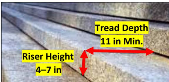
Figure 110: Riser and Tread Dimensions
