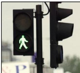
Figure 73: Pedestrian Signal Heads
