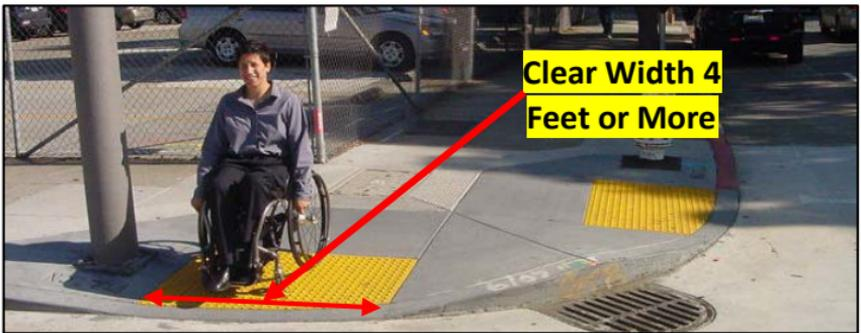
Figure 32: Curb Ramp Width
