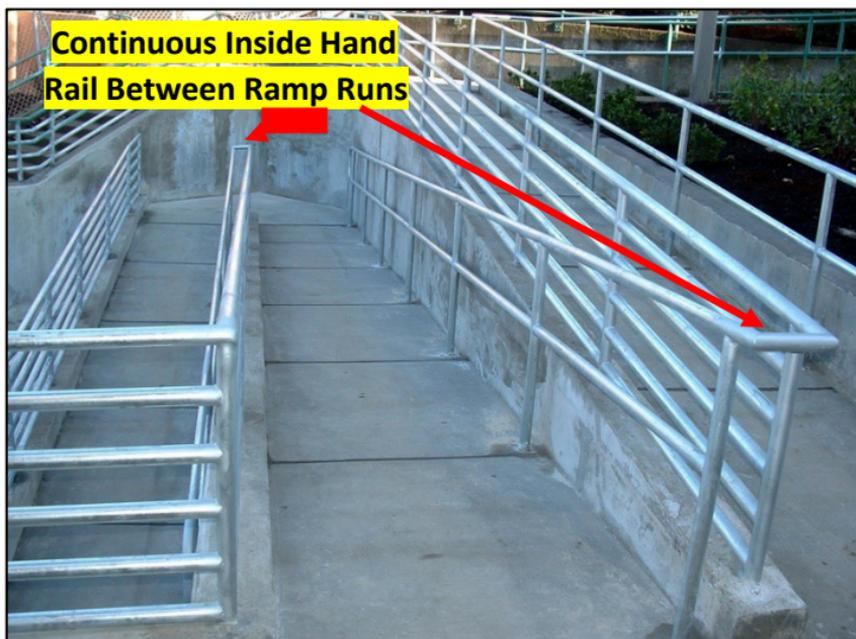
*Figure 113: Handrail Continuity Requirement*
