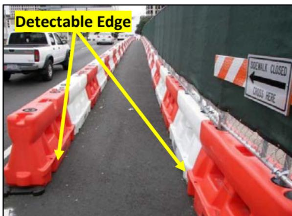
*Figure 31: Detectable Edge Provided Throughout the Length of the APAR*
