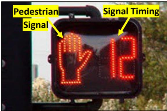
Figure 78: Pedestrian Signals Combined with Pedestrian Signal Timing
