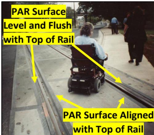
Figure 16: PAR Crossing Rails at Grade
