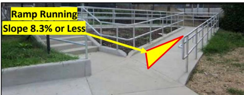
Figure 104: Ramp Running Slope
