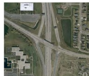
DIAMOND INTERCHANGE RAMP
