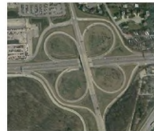
CLOVERLEAF INTERCHANGE RAMP
