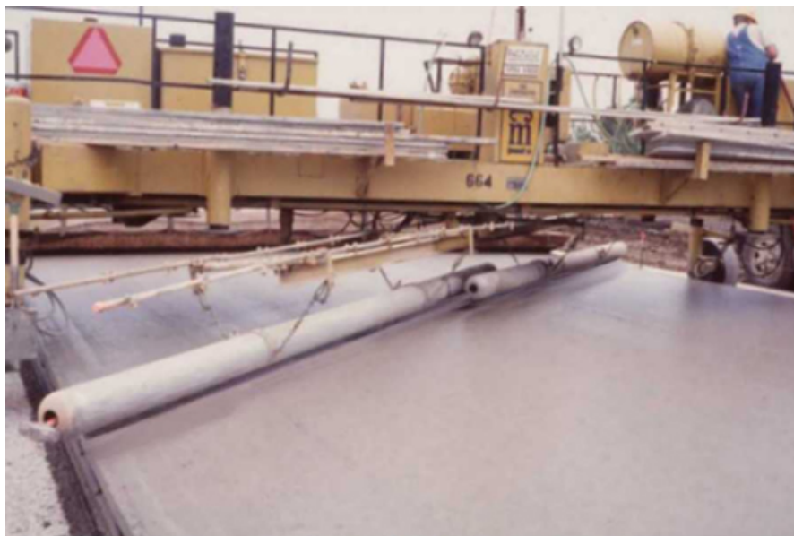
Figure 400-24 — TUBE FLOATING
