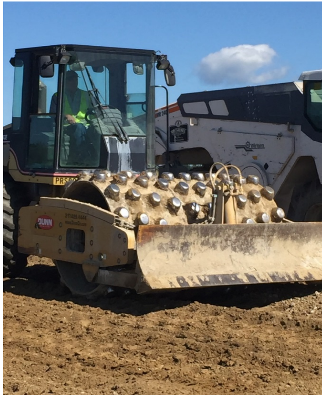
Figure 301-4 — SHEEPFOOT ROLLER ON SUBGRADE
