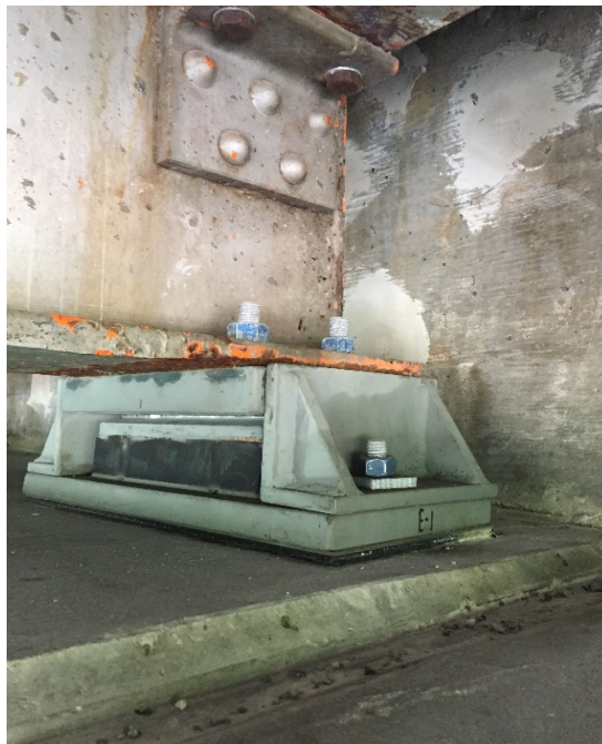
Figure 500-1 — ELASTOMERIC BEARING TYPE 2
