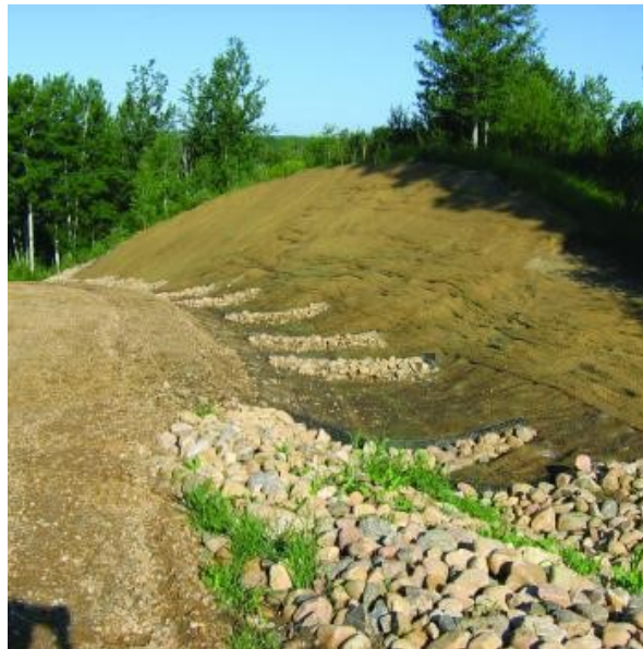
Figure 200-158 —AGGREGATE DITCH CHECK
