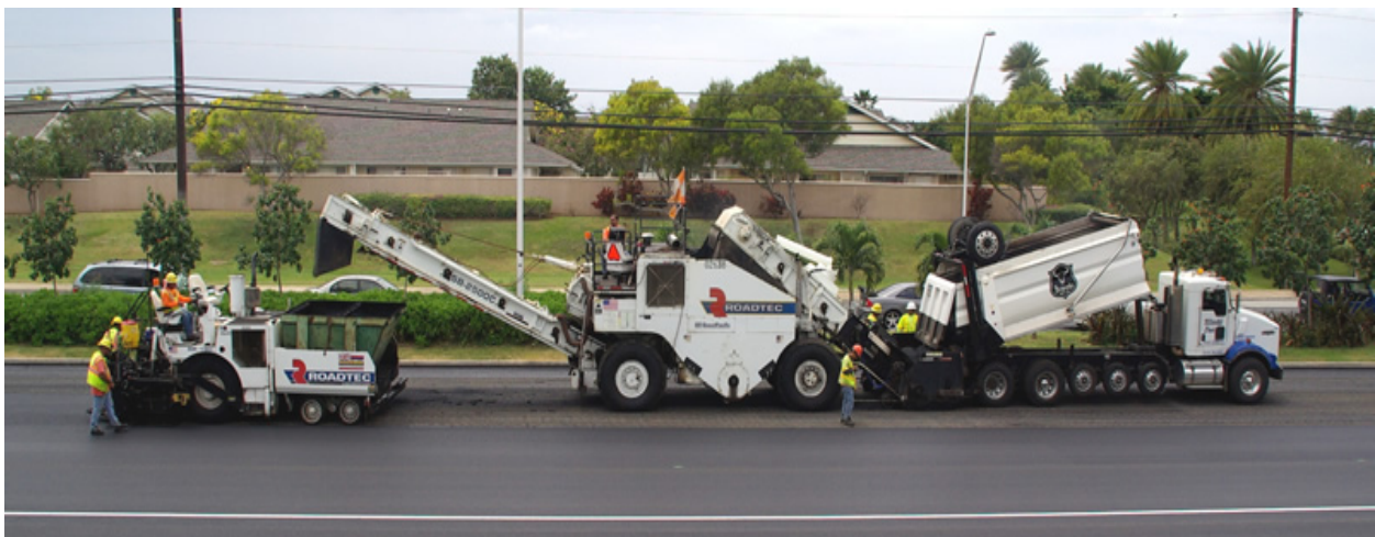
Figure 400-6 — PAVING TRAIN WITH MATERIAL TRANSFER DEVICE
