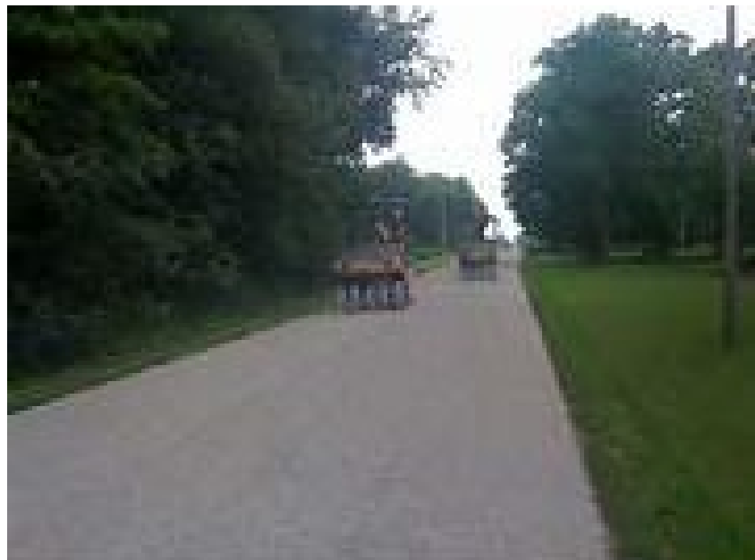
Figure 400-4 — ROLLING COVER COAT AGGREGATE WITH RUBBER-TIRED ROLLERS
