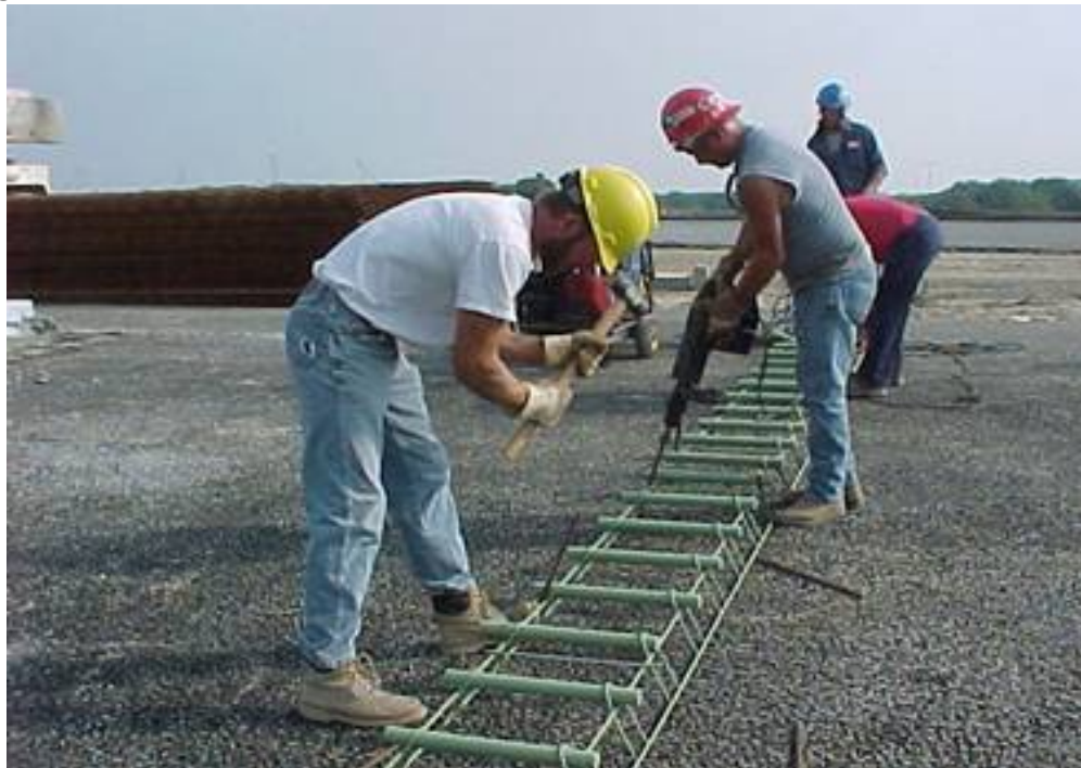
Figure 400-18 — DOWEL BASKET ASSEMBLIES ON AGGREGATE SUBBASE
