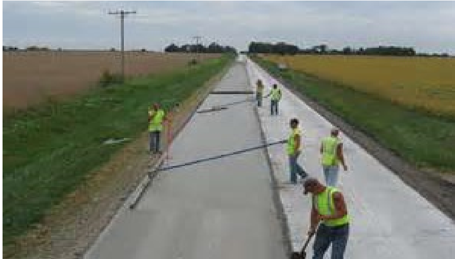
Figure 400-25 — FINISHING PCC CONCRETE PAVEMENT
