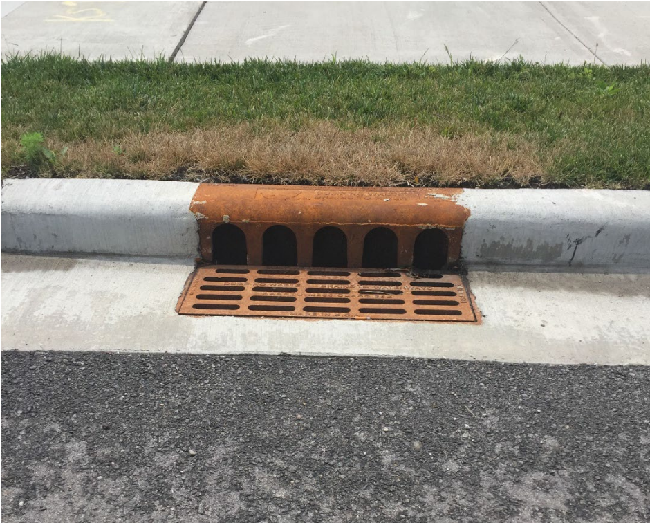
Figure 600-3 — TYPICAL FRAME AND GRATE FOR INLETS
