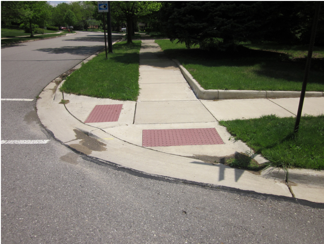
Figure 400-32 — ACCESSIBILITY-COMPLIANT CURB RAMP
