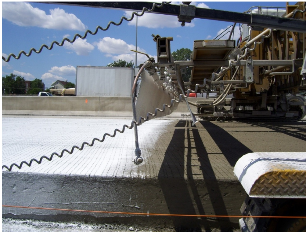
Figure 400-27 — MEMBRANE CURING FOR SLIPFORM PAVEMENT
