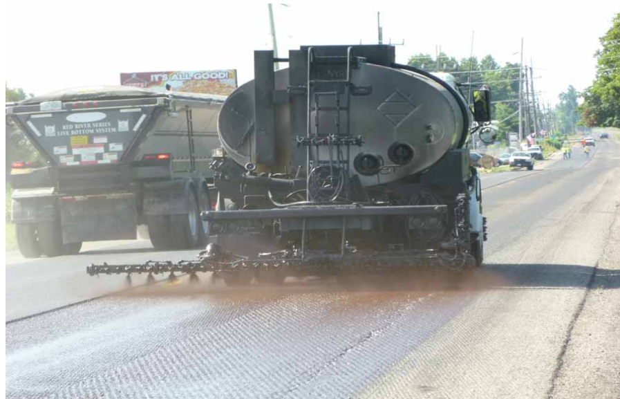
Figure 400-11 — APPLYING BITUMINOUS TACK COAT ON A MILLED SURFACE
