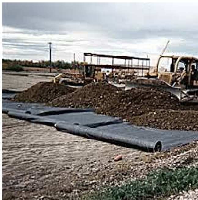
Figure 200-19 — FILTER FABRIC INSTALLATION
