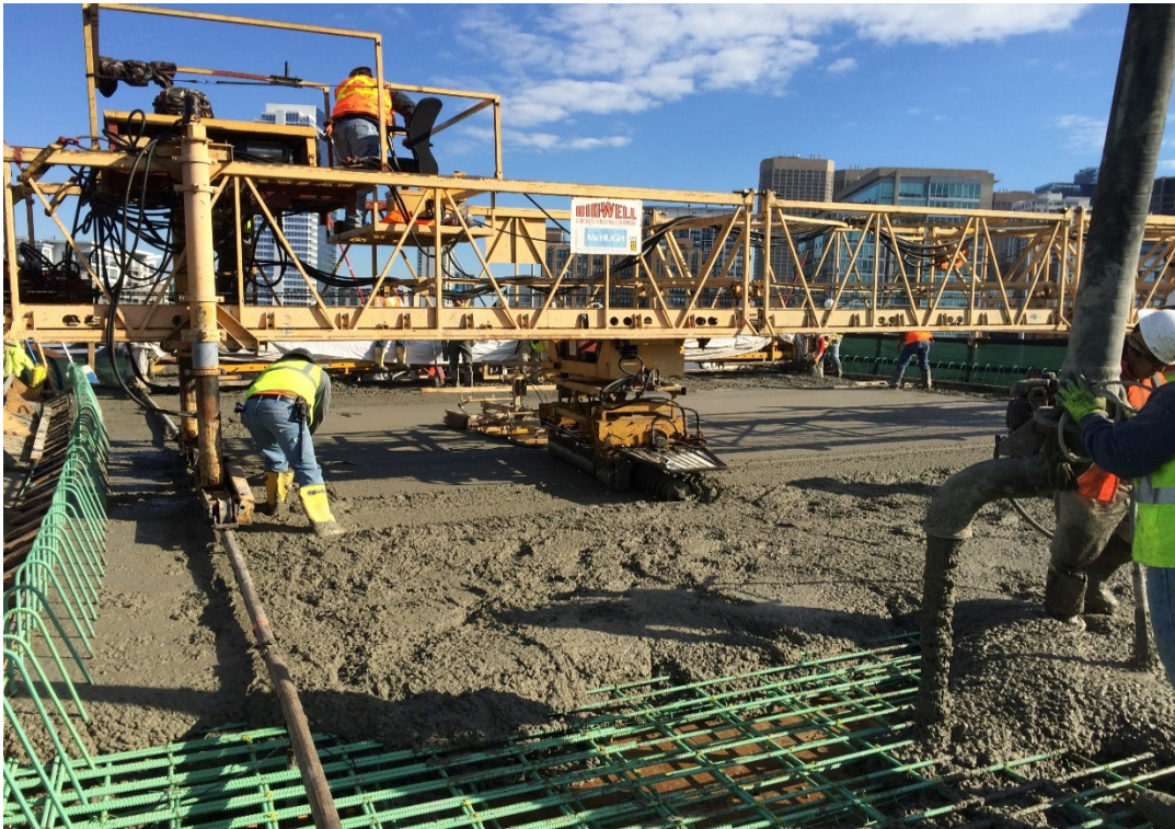
Figure 500-7 — BID-WELL DECK FINISHING MACHINE
