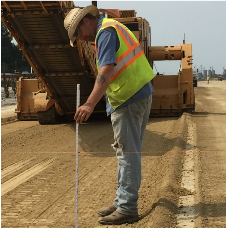
Figure 301-11 — CHECKING GRADE BEHIND TRIMMER
