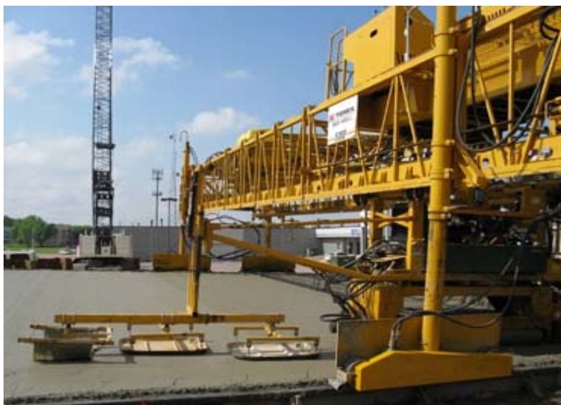
Figure 400-21 — CONCRETE FINISHING MACHINE RIDING ON SIDE FORMS
