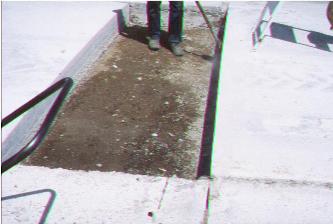
Figure 400-37 — CLASS D PATCHING
