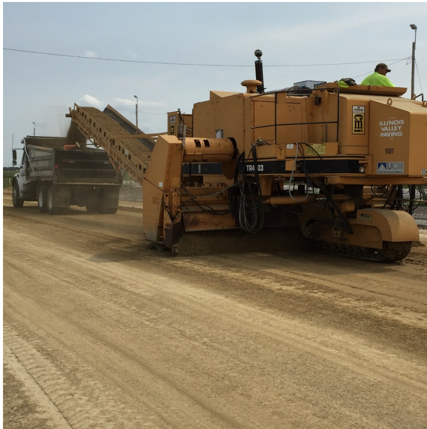
Figure 301-3 — BELT TRIMMER (Rough Trimming of Earth Subgrade)
