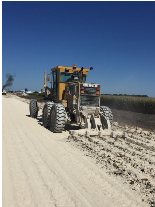
Figure 301-12 — SCARIFYING LIME TREATED SOIL
