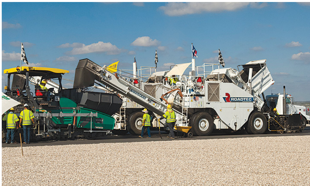
Figure 400-7 — PAVING TRAIN WITH MATERIAL TRANSFER DEVICE
