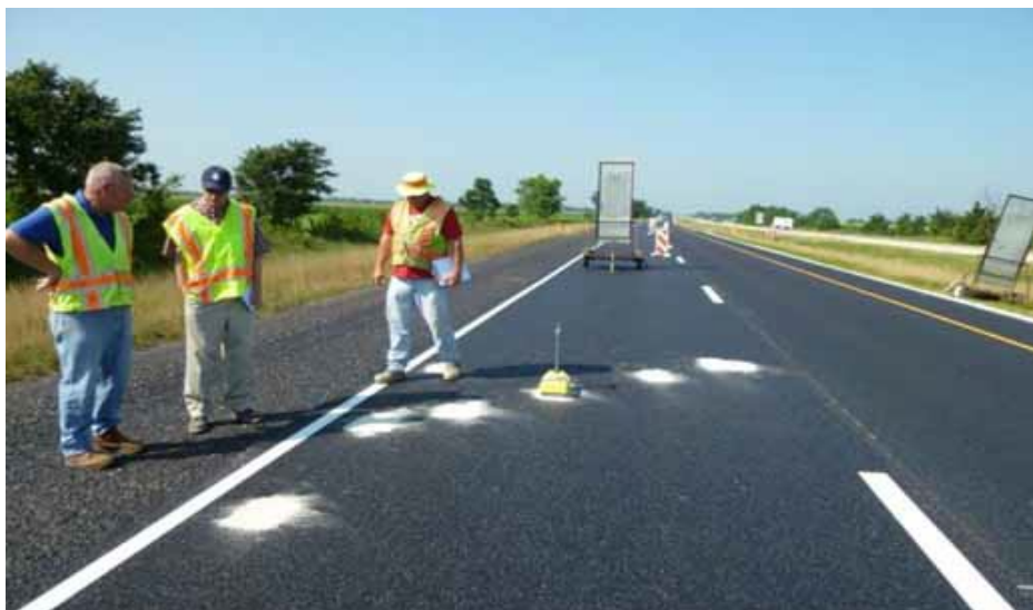
Figure 400-12 — DENSITY TESTING WITH A NUCLEAR GAUGE
