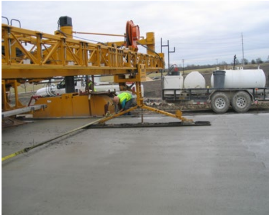
Figure 400-23 — MECHANICAL FLOATING
