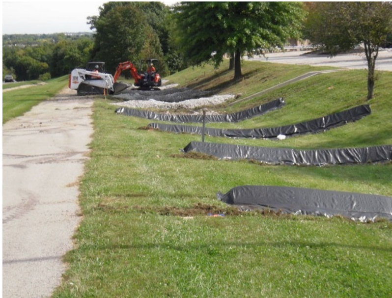
Figure 200-17 — GEOTECHNICAL DITCH CHECKS
