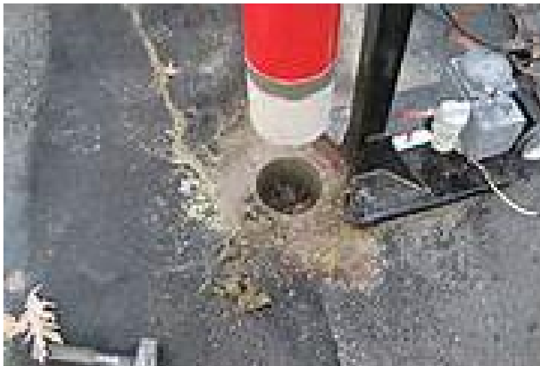
Figure 400-14 — CORING HMA PAVEMENT AT A RANDOM LOCATION
