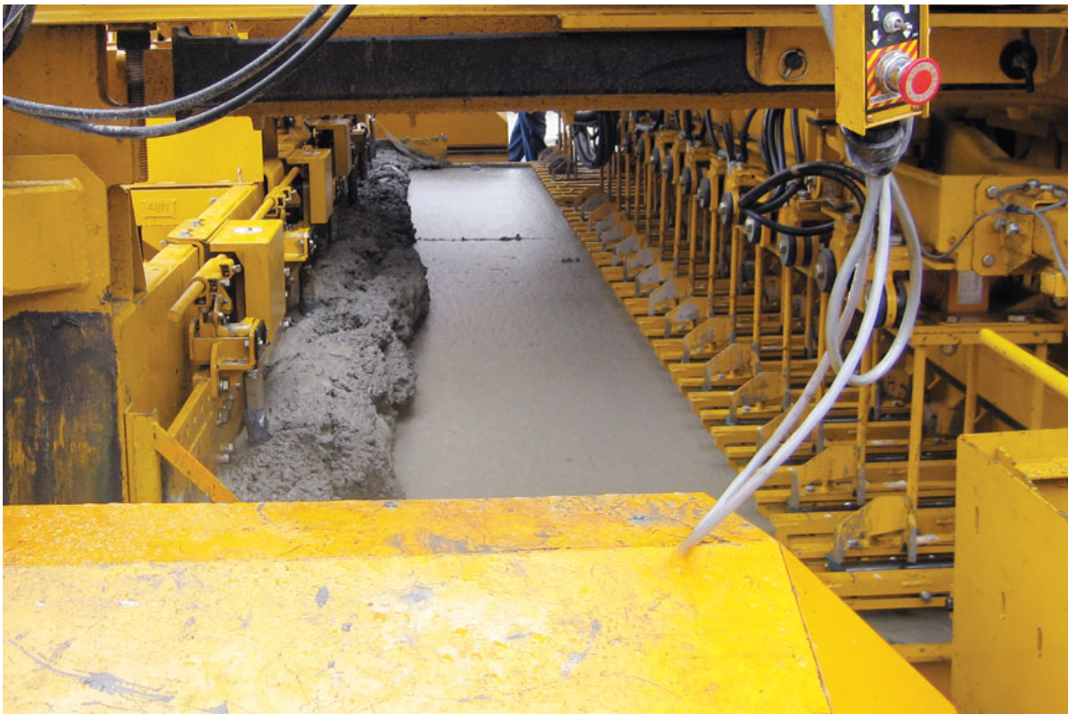
Figure 400-20 — CONCRETE PAVER WITH DOWEL BAR INSERTER (DBI)
