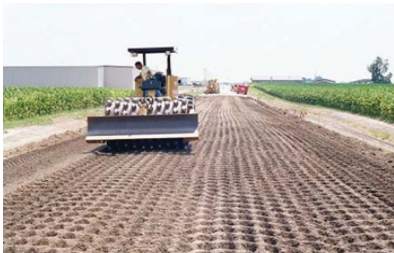
Figure 301-14 — SHEEPSFOOT ROLLER COMPACTING LIME TREATED SOIL
