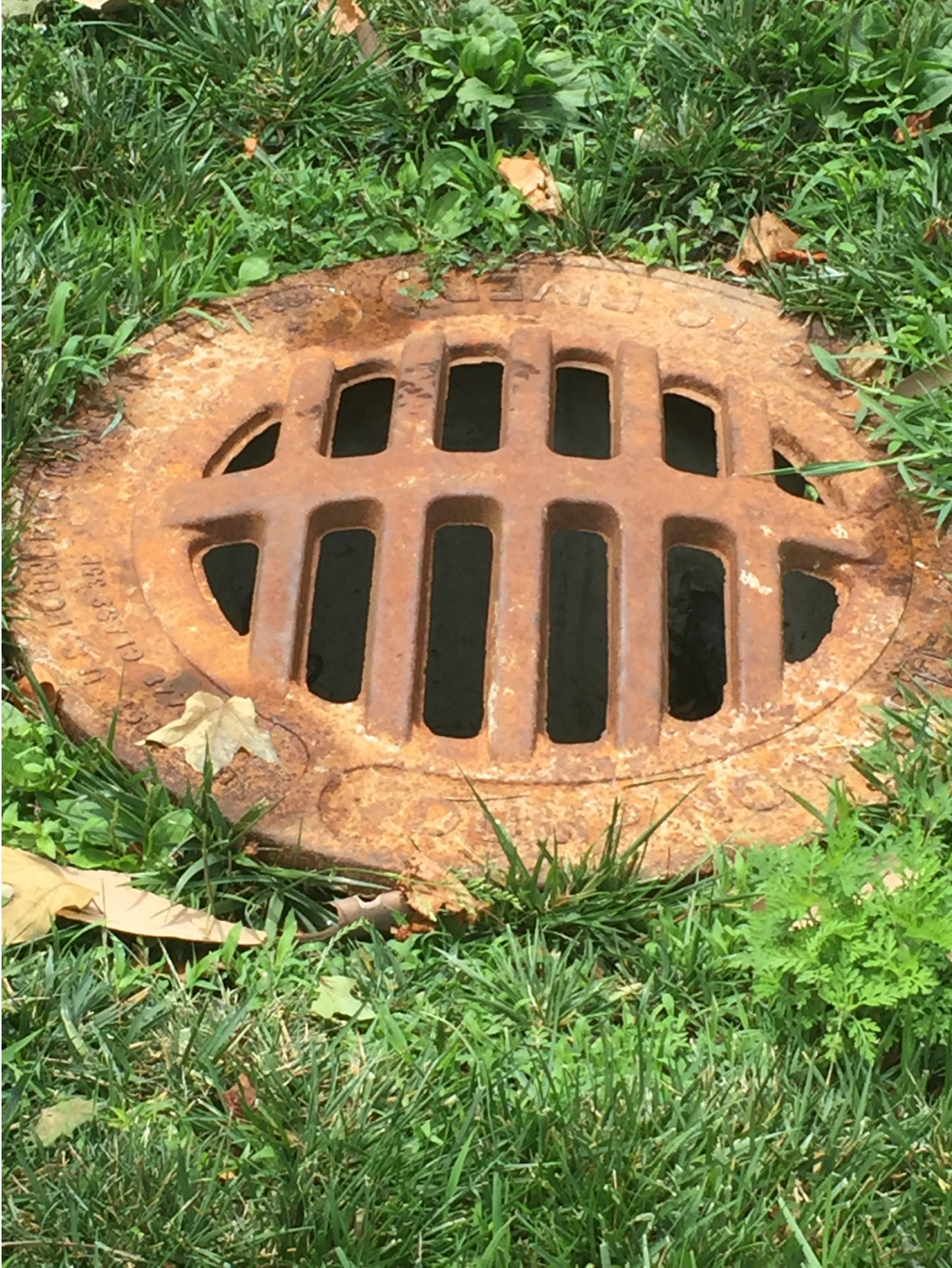
Figure 600-2 — TYPICAL FRAME AND GRATE FOR CATCH BASINS
