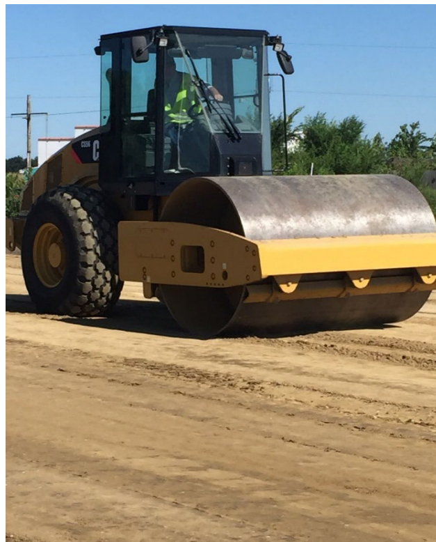
Figure 301-5 — STEEL WHEEL ROLLER ROLLING SUBGRADE
