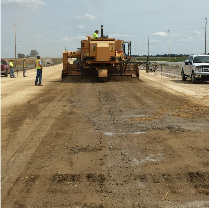
Figure 301-10 — SUBGRADE MACHINE (Final Trimming of Earth Subgrade)
