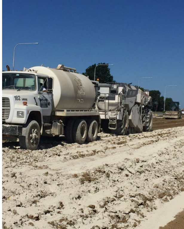
Figure 301-13 — MIXING LIME WITH SOIL WITH A ROTARY SPEED MIXER
