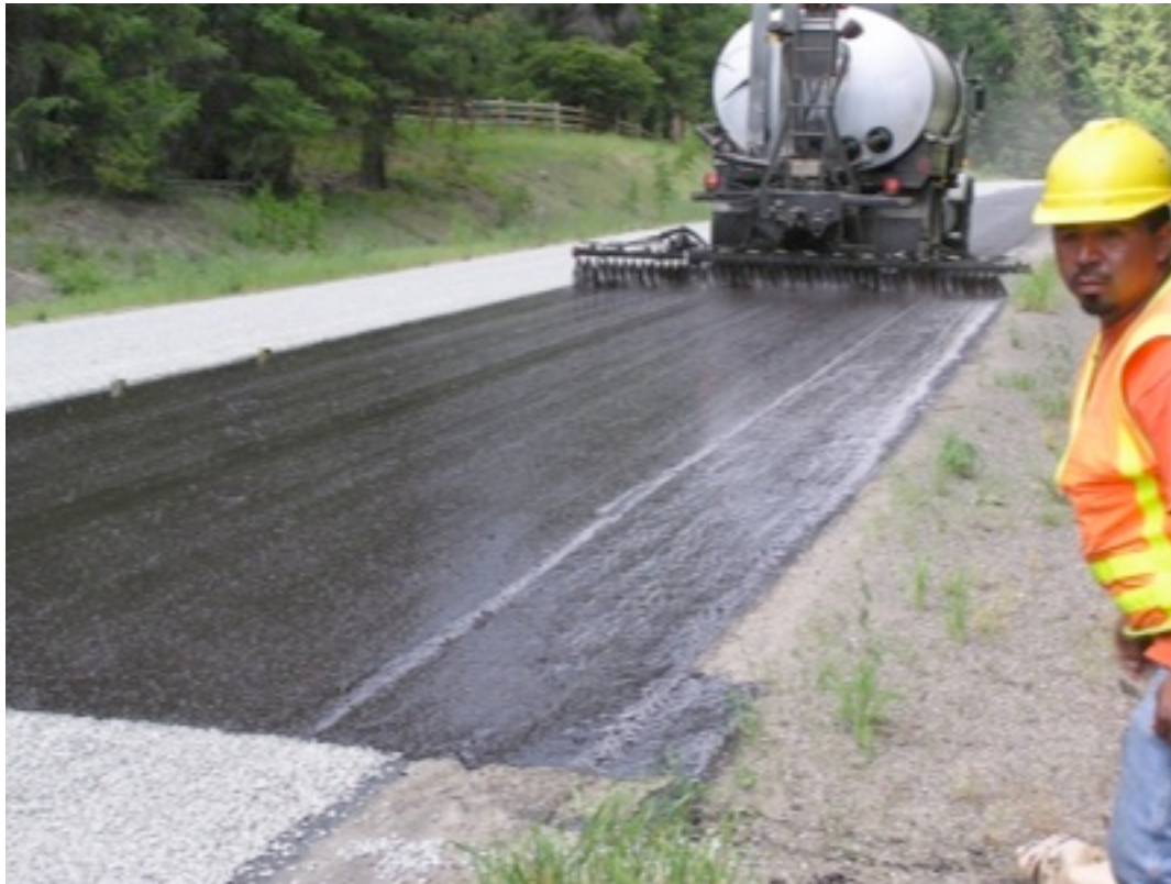
Figure 400-2 — DISTRIBUTOR TRUCK APPLYING PRIME COAT
