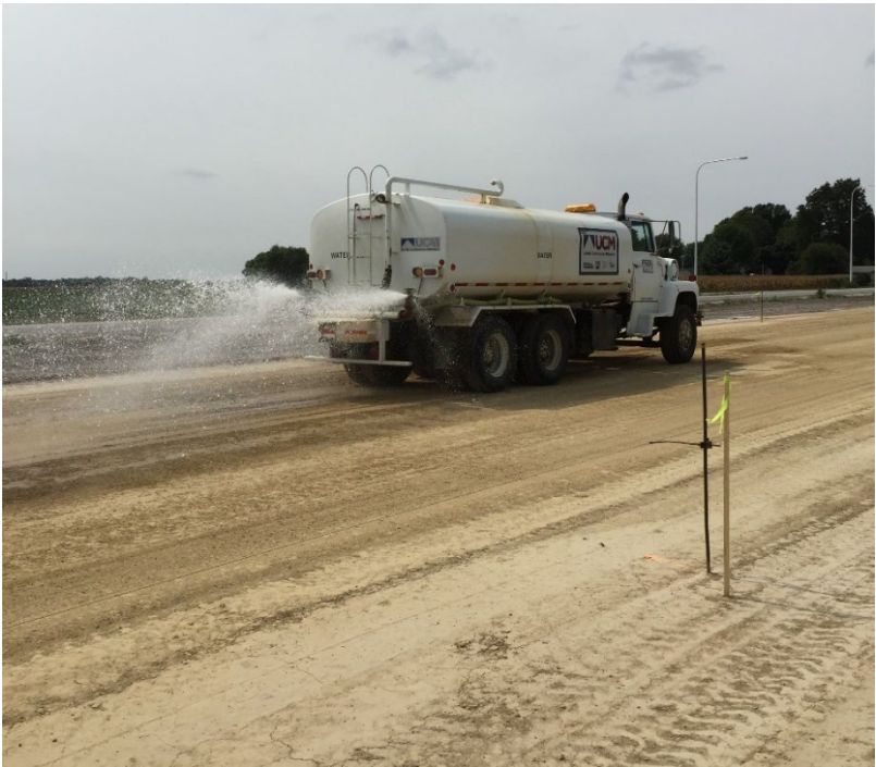
Figure 301-9 — WATER TRUCK WATERING SUBGRADE (Prior to Trimming)
