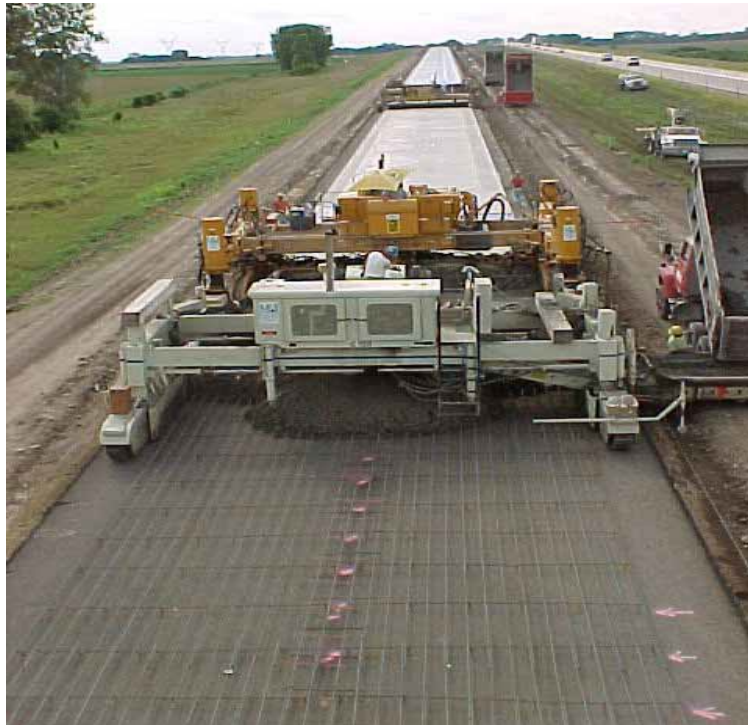
Figure 400-31 — CRCP PAVING
