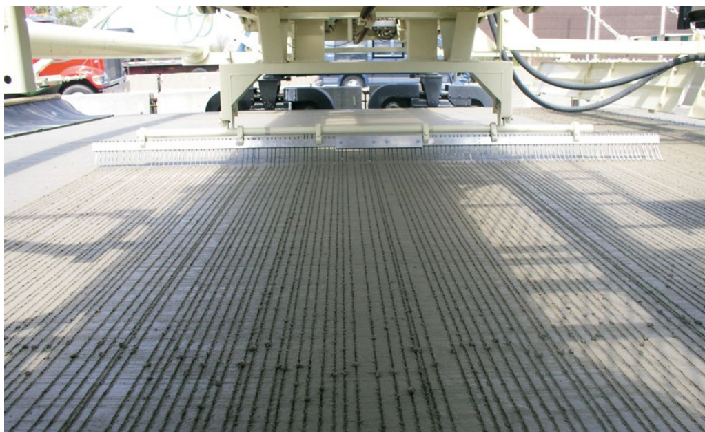
Figure 400-26 — TINING PCC PAVEMENT WITH RANDOM SPACING
