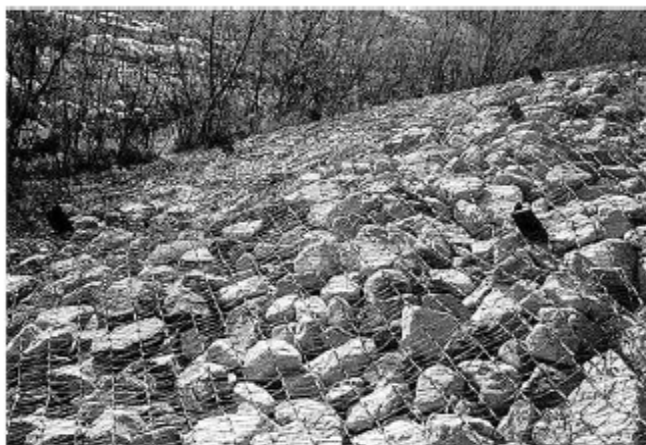
Fig. 11-102.023 1 Wire enclosed riprap used for slope protection
