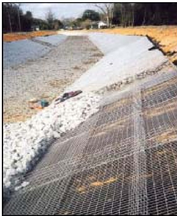
Fig. 11-102.022 1 Field installation of gabion mattress on streambank
