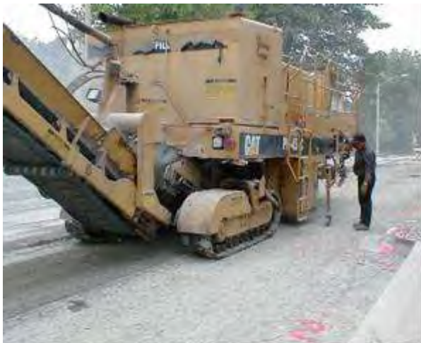
Step 1 & 2. Pre-overlay repair & milling and cleaning. Localized areas of distress are repaired prior to overlay placement. The surface is milled to remove rutting and restore profile prior to PCC placement.
