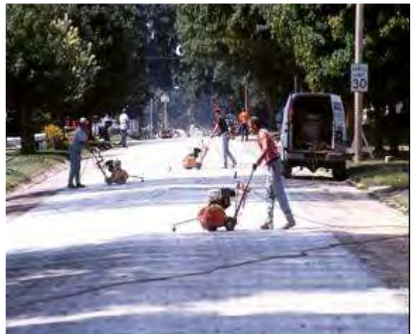
Step 5. Joint sawing & curing. Timely joint sawing is required to establish the contraction joints in the PCC pavement. Curing is important for UTW overlays due to the high surface-area-to-volume ratio.
