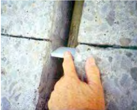
Step 5. Caulking the joint/crack. The joint/crack edges are caulked to stop the flow of material from the slot.
