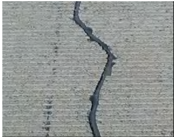
Step 4. Application of sealant. The last step is to place the sealant in the refaced crack per governing specifications.
