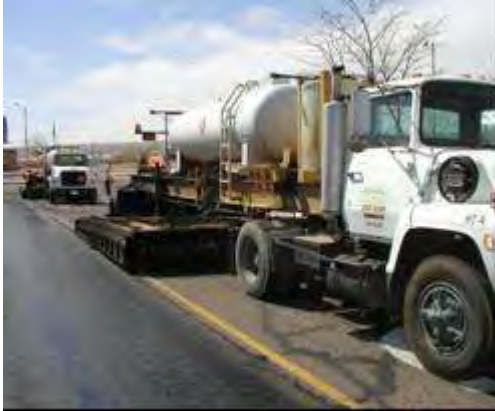
Step 1. Heating the surface. The surface is heated to soften the existing material.
