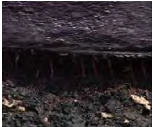
Step 3. Addition of Rejuvenator. A rejuvenating agent is sprayed onto the loosened material and mixed.
