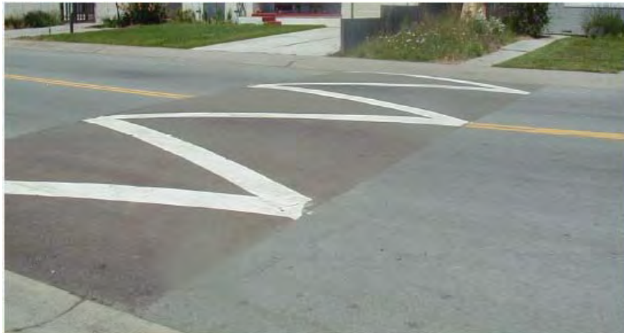
Figure 9-8. Speed humps are a common vertical measure for controlling the speed of motorists in residential neighborhoods.
