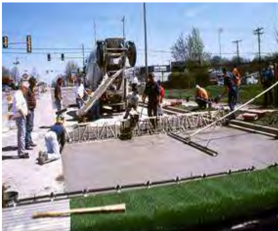
Step 4. Finishing & texturing. The PCC is finished and textured using conventional methods.
