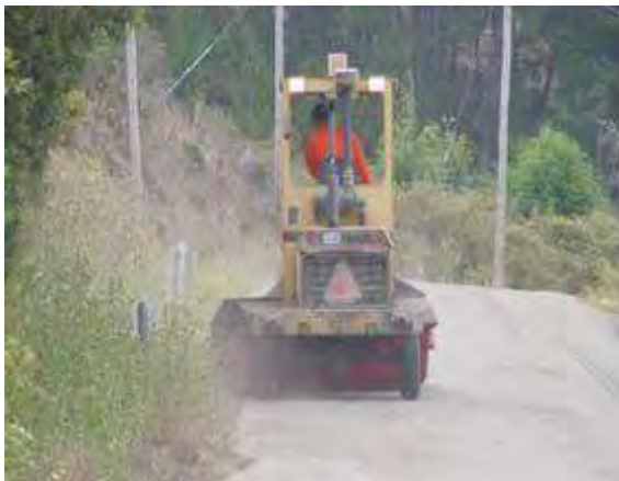
Step 1. Surface preparation. Surface must be clean and dry to ensure good bond with the asphalt.
