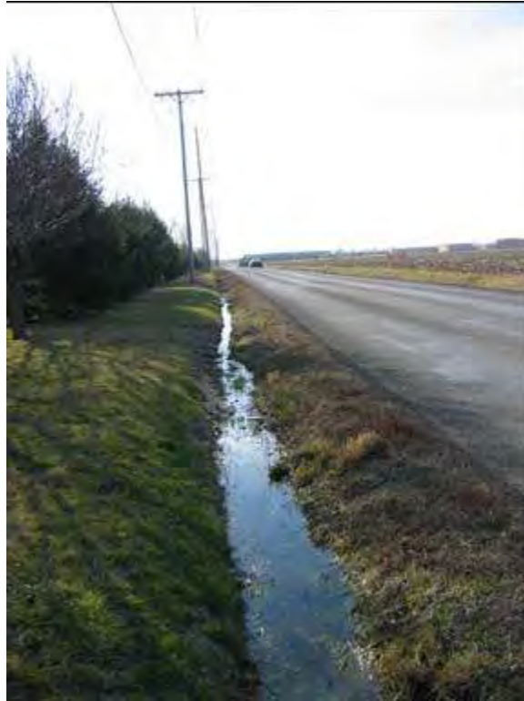
Drainage Preservation. This photo shows an example of a ditch with obstructed flow.
