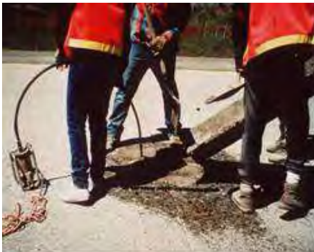
Step 7. Repair material placement. Material should be placed per governing specifications.
