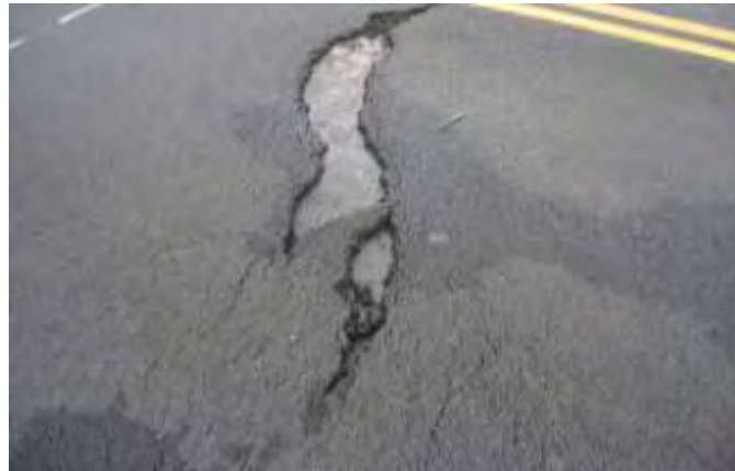
SLIPPAGE CRACKING
