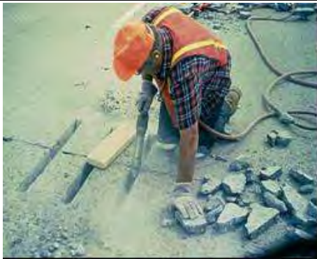
Step 1 & 2. Slot creation and material removal. Slots are cut and concrete material is removed.
