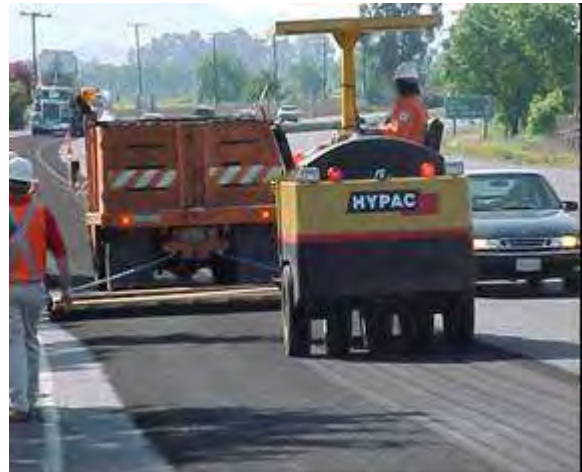
Steps 4 & 5. Drag-brooming of sand and rolling. After the application of sand, the surface is drag-broomed again and rolled with pneumatic-tired rollers.
