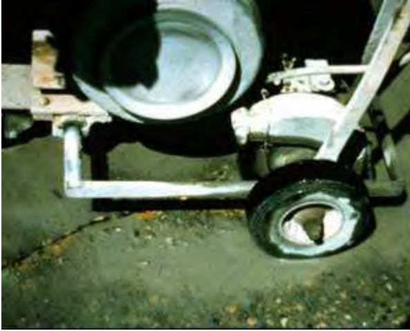
Step 1. Crack refacing. Small crack saws are used to reface cracks and create a reservoir for the sealant.
