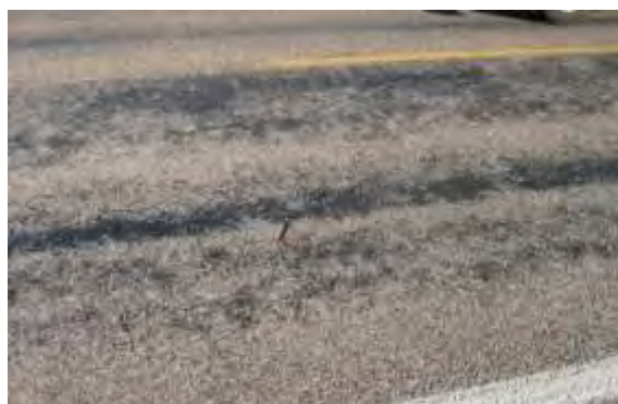
Moderate Bleeding – Bleeding is apparent over large or continuous areas of the pavement surface.
