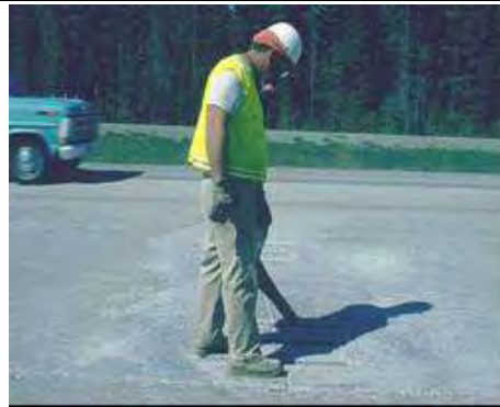
Step 3 & 4. Sandblasting and cleaning. Slots are sandblasted and cleaned in preparation for dowel bars.
