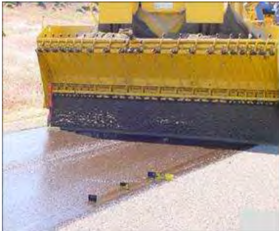
Step 3. Sand application. A thin layer of sand is applied to the broomed emulsion.
