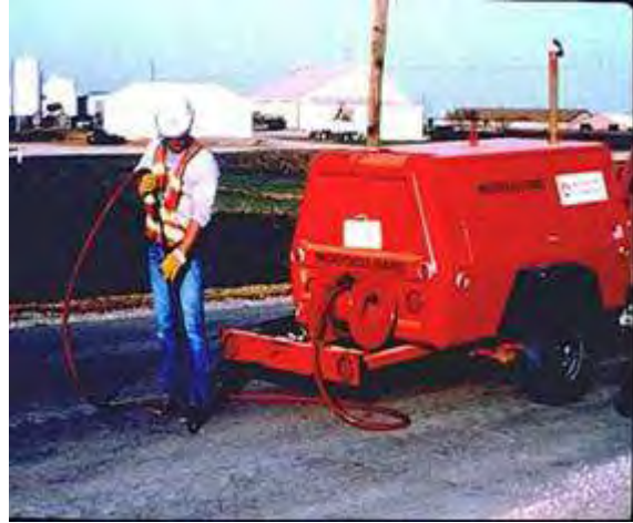
Step 2. Cleaning. Cracks must be clean and dry to enhance sealant bonding.
