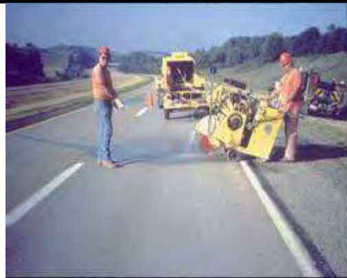
Step 2. Concrete removal. Sawing the boundaries and removing deteriorated PCC.
