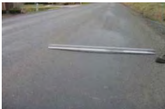
Light Rutting - Rut depth visible, approximately less than ½ inch (12.7 mm) in a given location.
