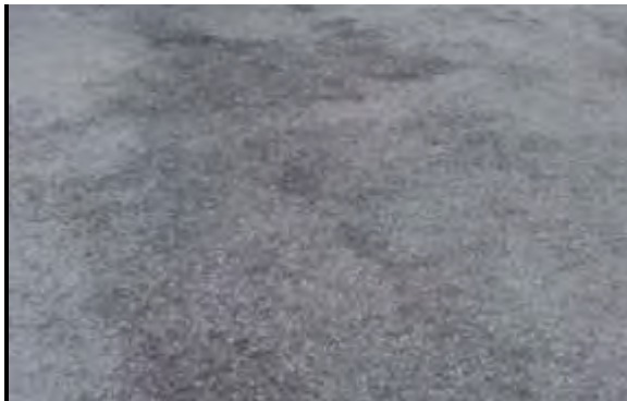
Severe Weathering/Raveling - Considerable aggregate loss resulting in an overall rough pavement surface with pitted/eroded areas.
