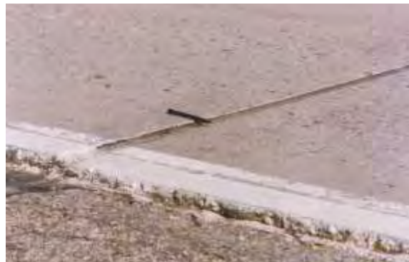
Moderate Faulting - Faulting measures approximately ¼ inch to ½ inch (6.4 mm and 12.7 mm) at a given location.
