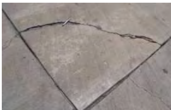
Moderate Corner Breaks - Crack has some spalling and the corner piece is intact and has little or no movement under load.
