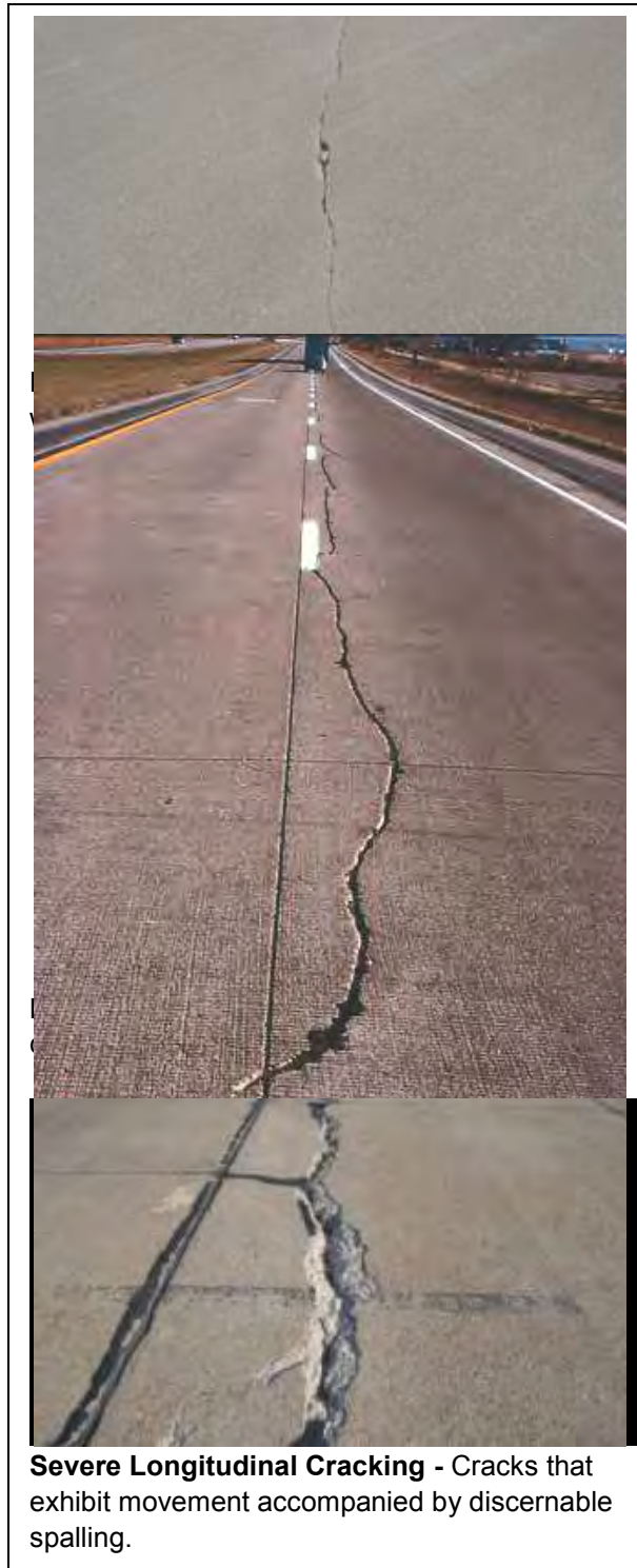
LONGITUDINAL CRACKING SEVERITY LEVELS
