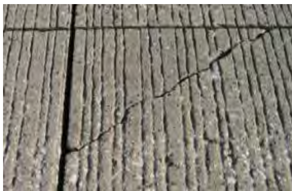
Light Corner Breaks - Crack is hairline and unspalled; the resulting corner piece is not cracked or shows no movement under load.
