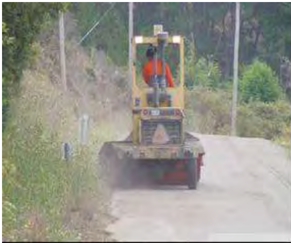
Step 1. Surface preparation. The surface must be free of dust, dirt, and debris prior to applying the emulsion.
