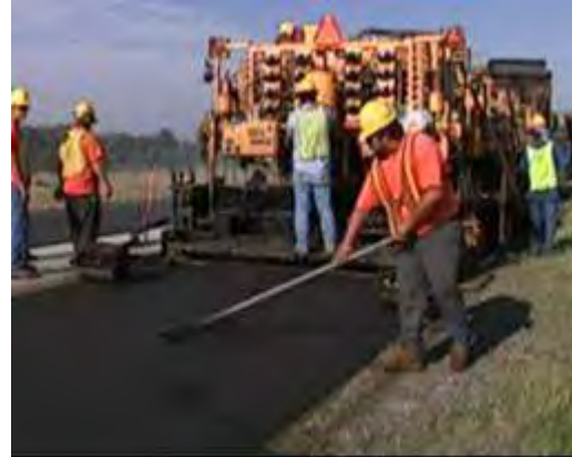
Step 4. Laydown. Mixed material is placed with conventional equipment.
