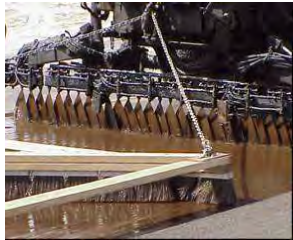
Step 2. Emulsion application and drag-brooming. Drag-brooming is used to work emulsion into cracks and surface voids.
