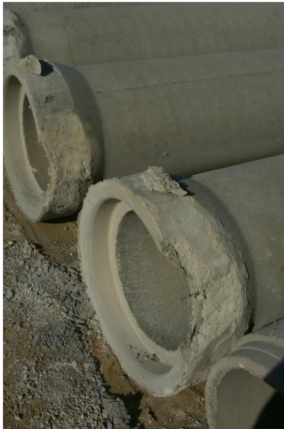
Figure 24 - Broken Bell – Too Large to Repair
