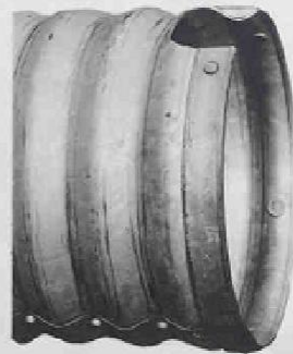
Figure 13 - Galvanized Bar Satisfactory
