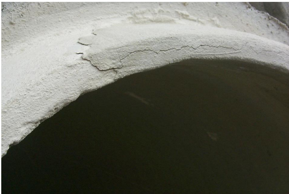
Figure 14 - Unacceptable Patch
