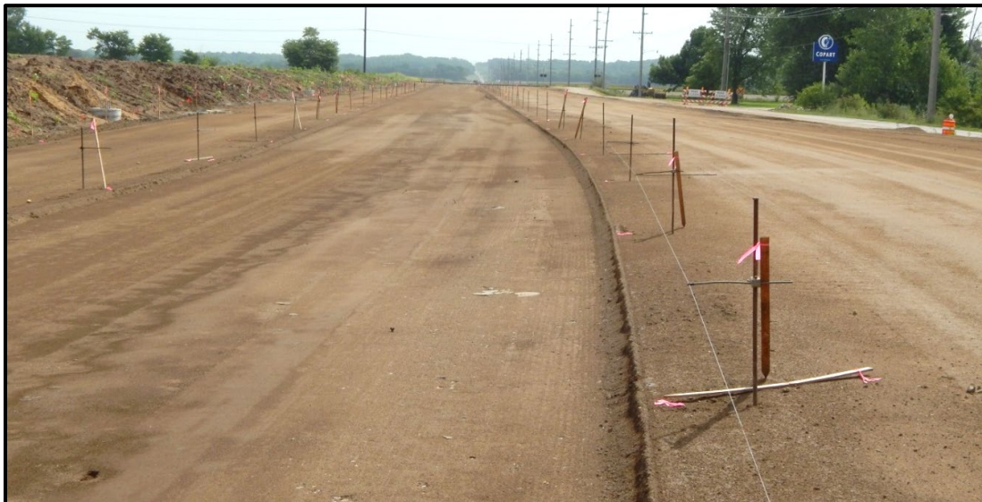
Figure 15. Photo of Fly ash modified Improved Subgrade is fine graded and ready for paving.
