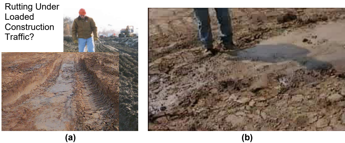
Figure 18. Photos of rutting (a) and pumping (b) under proof rolling or construction traffic.
