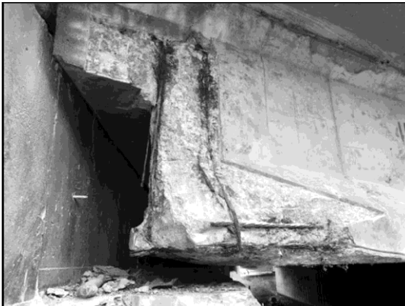
BEAM DAMAGE
