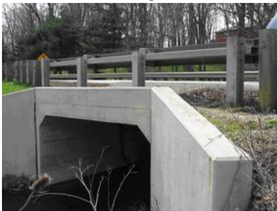
OH Type 5 Nested W-Beam/Tubular Culvert Rail
