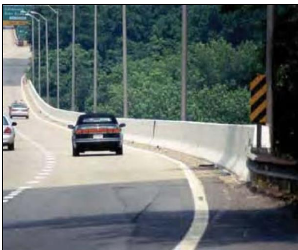
Type: 42" Tall Concrete Safety-Shaped Bridge Railing Source: 2011 AASHTO Roadside Design Guide Fig 7-5 Code: M095
