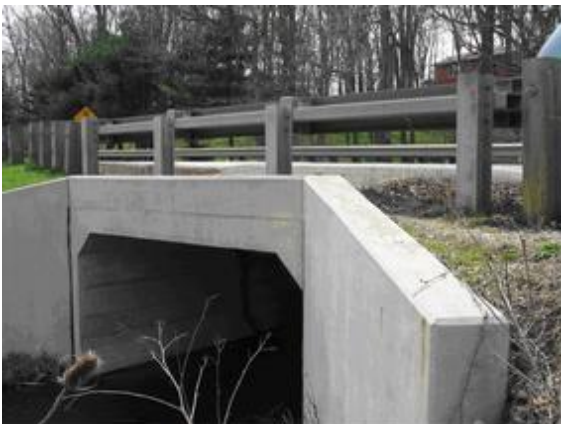
OH Type 5 Nested W-Beam/Tubular Culvert Rail
