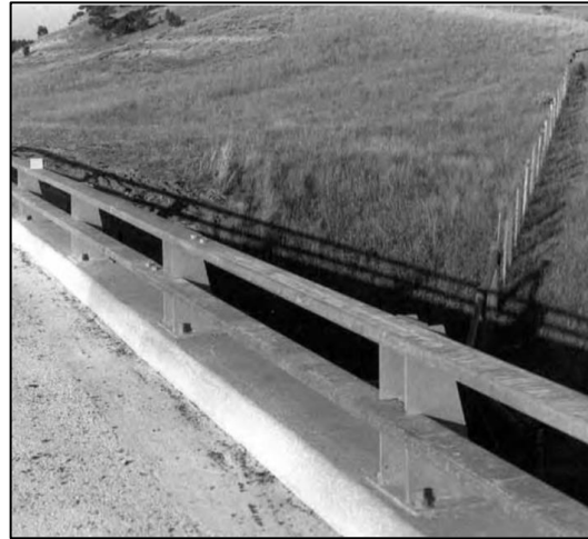
Type: Wyoming Two-Tube Bridge Railing
