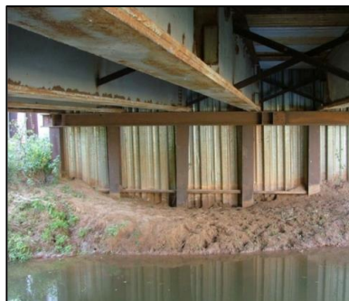
A08 Pile bent with lagging:
