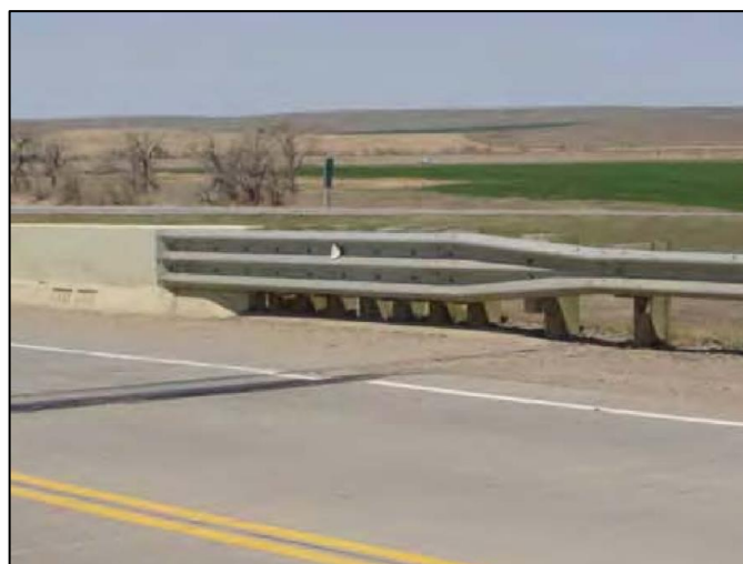
Type: Thrie-Beam Transition to Modified Concrete Safety Shape Source: 2011 AASHTO Roadside Design Guide Fig 7-12 Code: 3503
