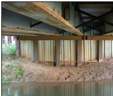
A08 Pile bent with lagging:
