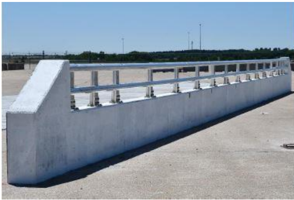
NC Two-Bar Metal Bridge Rail
