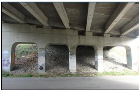
B01 Bent column or open, or P03 Pier multiple column:
