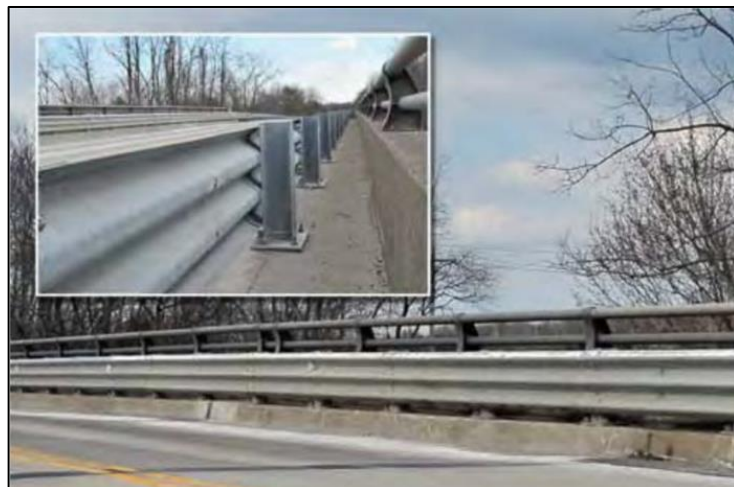
Type: Delaware Thrie-Beam Retrofit Source: 2011 AASHTO Roadside Design Guide Fig 7-10 Code: 3504
