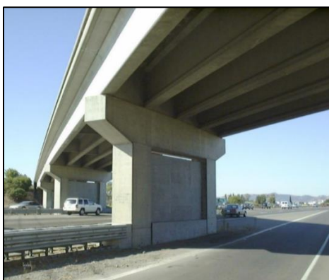
B02 Bent column w/ webwall, or P04 Pier multi column w/ webwall:
