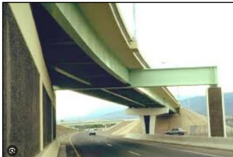
B04 Bent – straddle or c-shaped, or P05 Pier – straddle or c-shaped
