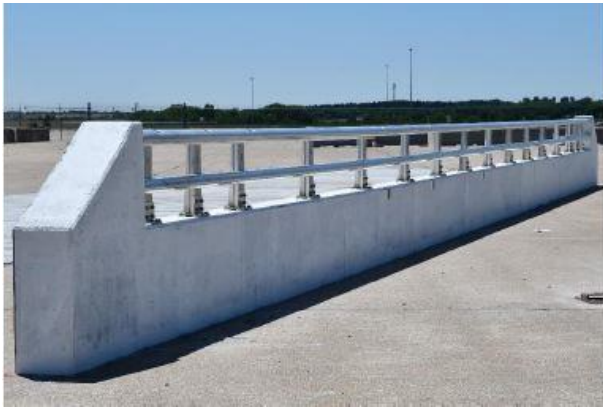
NC Two-Bar Metal Bridge Rail
