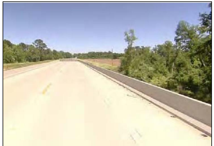
Type: Concrete F-Shaped Bridge Railing
