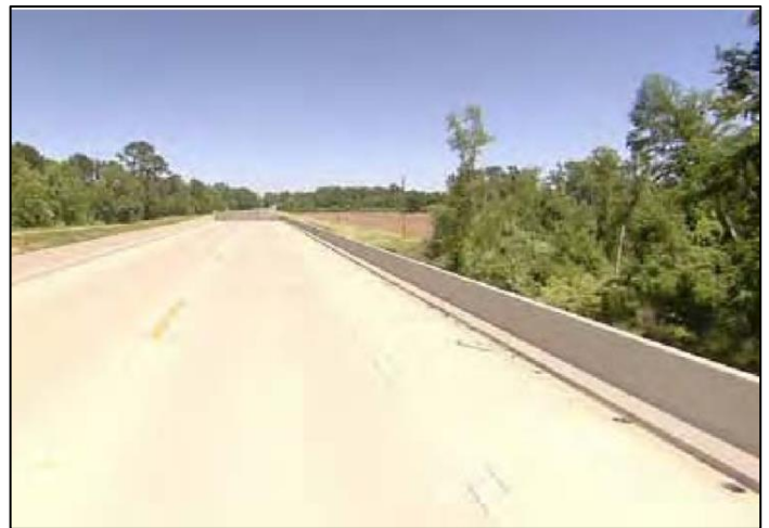
Type: Concrete F-Shaped Bridge Railing
