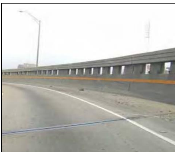
Type: Texas Type TT Railing Source: 2011 AASHTO Roadside Design Guide Fig 7-6 Code: M096
