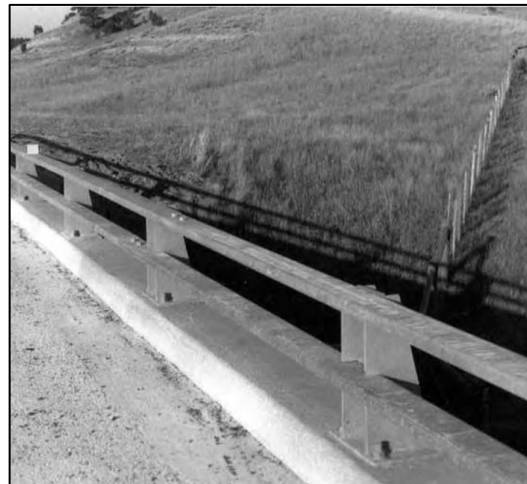
Type: Wyoming Two-Tube Bridge Railing
