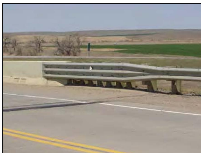
Type: Thrie-Beam Transition to Modified Concrete Safety Shape Source: 2011 AASHTO Roadside Design Guide Fig 7-12 Code: 3503
