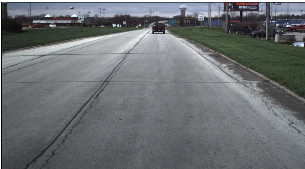
Figure 1-1.4-2 - Good Pavement
