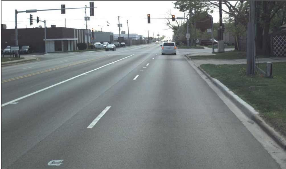
Figure 1-1.4-1 - Excellent Pavement
