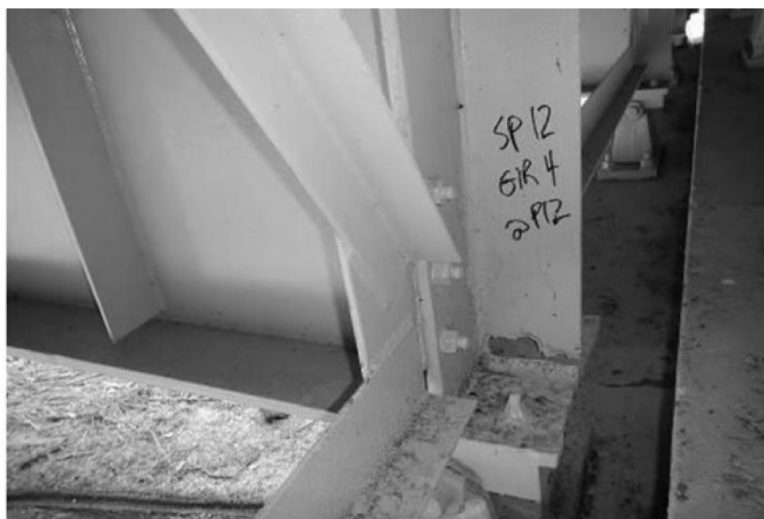
PICTURE 71 SN xxx-xxxx Date xx/xx/xxxx Girder 4 Span 12, Pier 12, East Bearing Bottom of girder web Full section loss Looking Southeast
