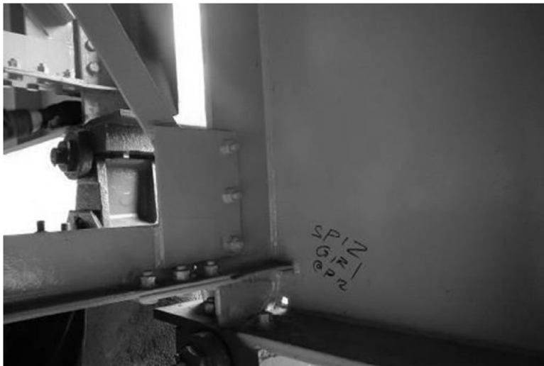
PICTURE 69 SN xxx-xxxx Date xx/xx/xxxx Girder 1 Span 12, Pier 12, East Bearing Bottom of web/stiffener Full section loss Looking Northwest
