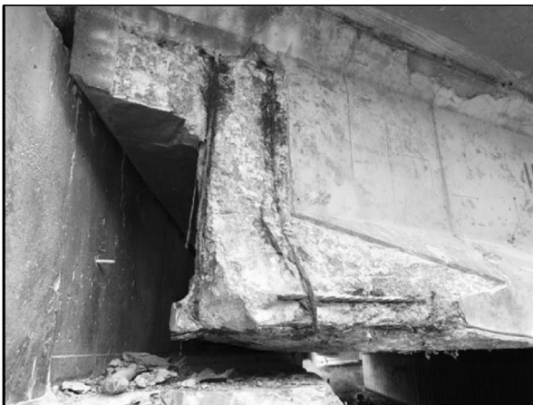
BEAM DAMAGE
