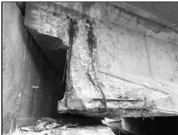
BEAM DAMAGE
