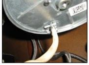
Check the kitchen stove anti-tip device. Owner must install the antitipping anchor for stoves according to the manufacturer's
